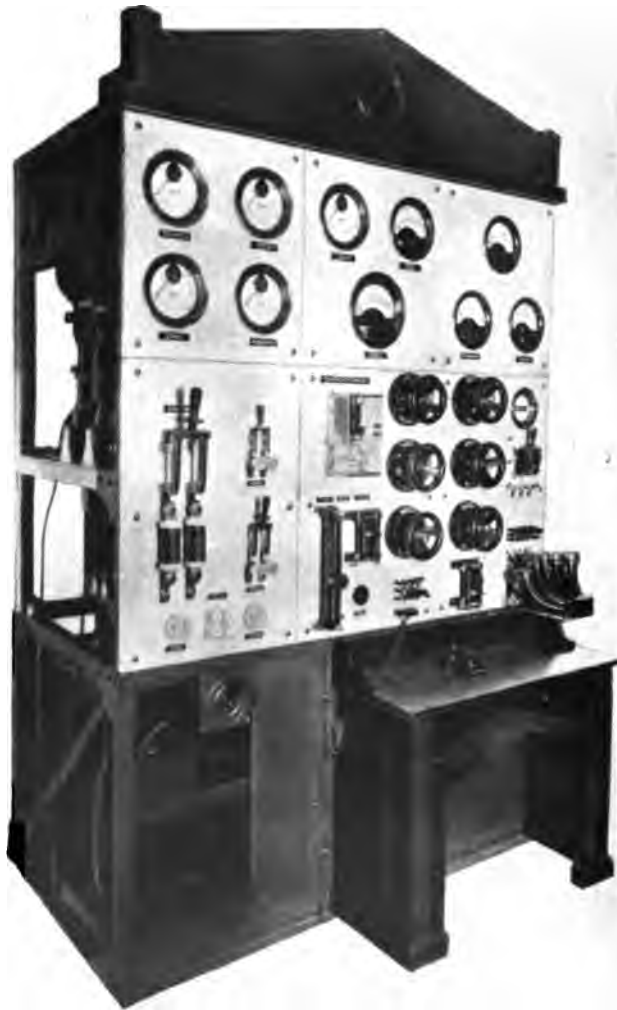
FIG. 195.—Wireless telephony installation on board the "Waterland," 1914.
